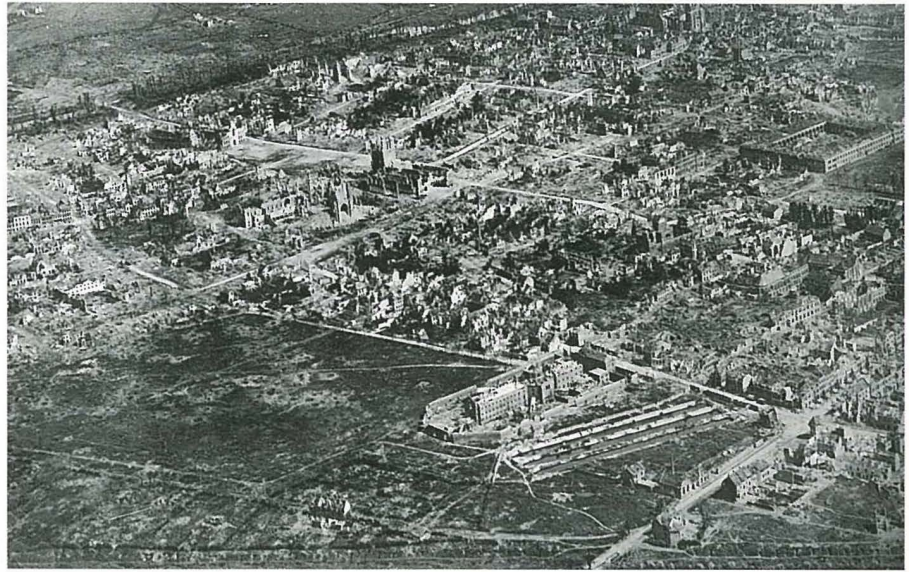
An aerial photograph of Ypres in Belgium showing the almost complete destruction of the town by four years of heavy gun bombardment.
